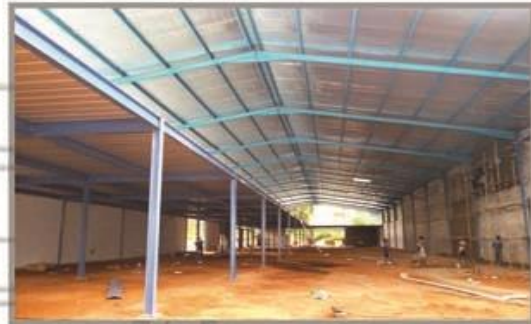
Decking & Clading work at Maspotha
